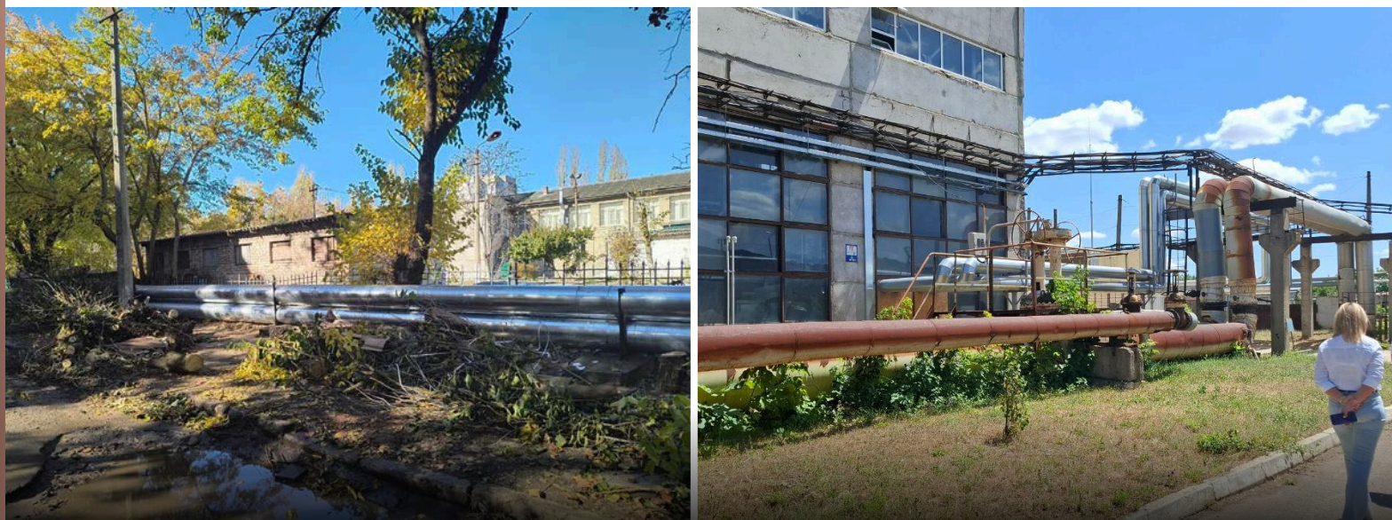
Thermal insulation in Mykolaiv: some areas already have new insulation, others are planned for replacement.
