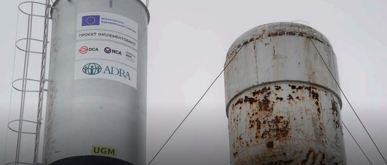
Installation of a water tower in the village of Pervomayske, Mykolaiv region
